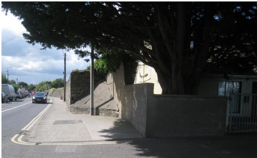
Fig.6: Non-historic section of entrance wall at the southeast of the site, proposed for demolition.
