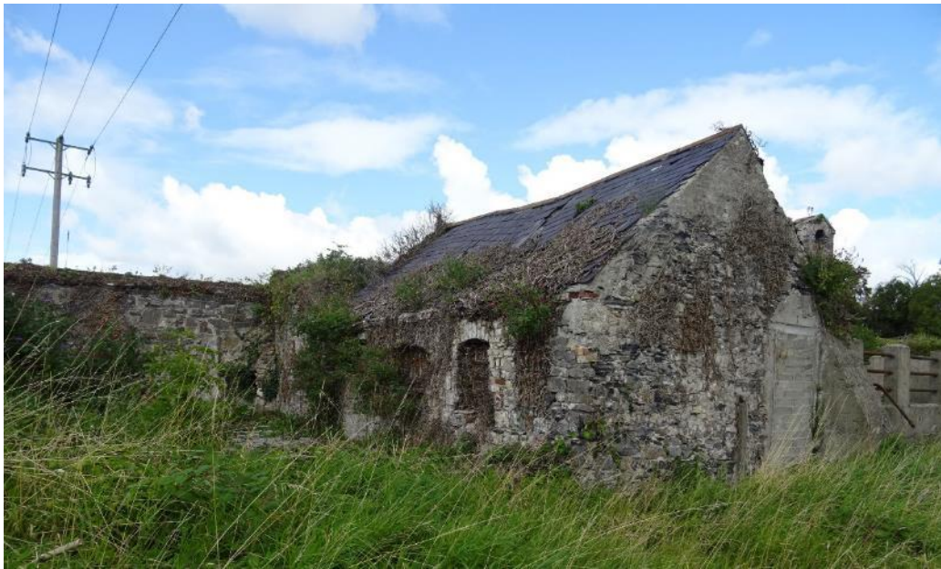
Fig.5: Historic Farm building proposed for demolition.
