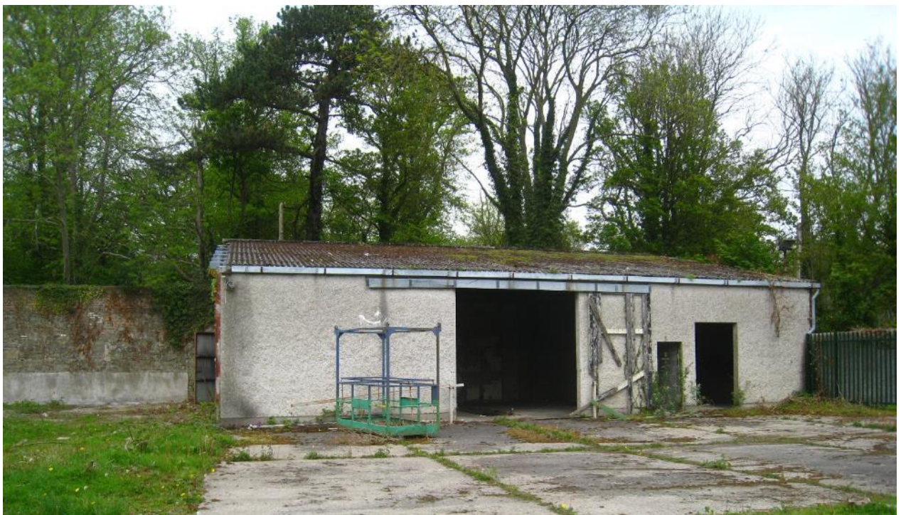
Fig.11: Non-historic ancillary building at the south of the north walled garden, proposed for demolition.
