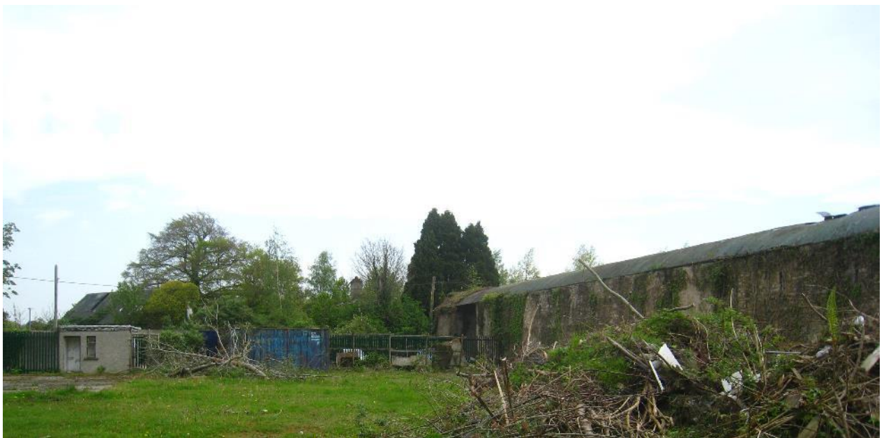
Fig.13: Non-historic ancillary building at the north of the Coach House, proposed for demolition.
