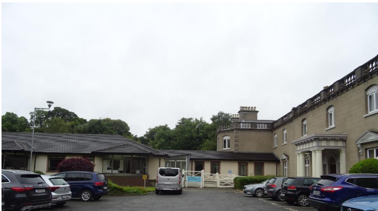
Fig.14: Non-historic 1980s ward extension at the south of St. Edmundsbury House, proposed for demolition.
