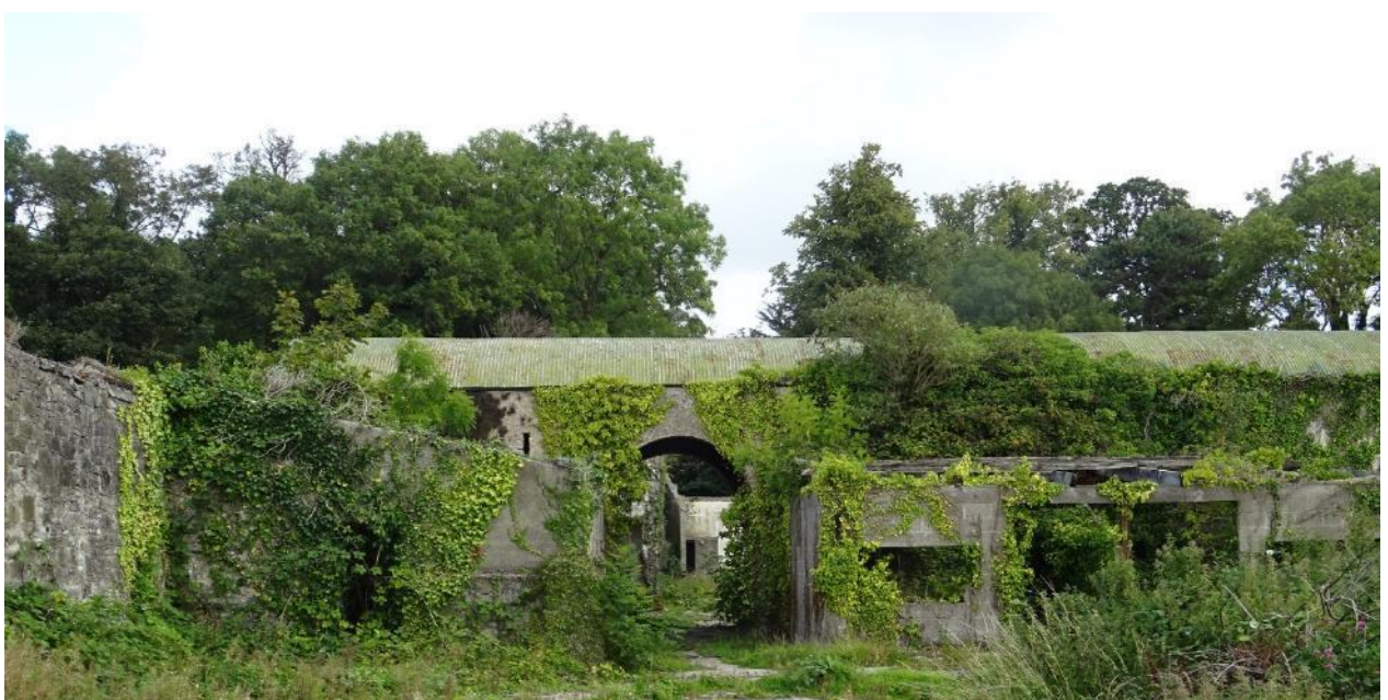
Fig.9: Non-historic concrete blocks outbuildings at the southeast of the Coach House, proposed for demolition.
