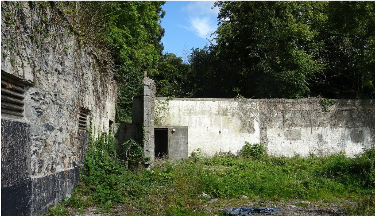
Fig.12: Non-historic ancillary building close to the Barn, proposed for demolition.
