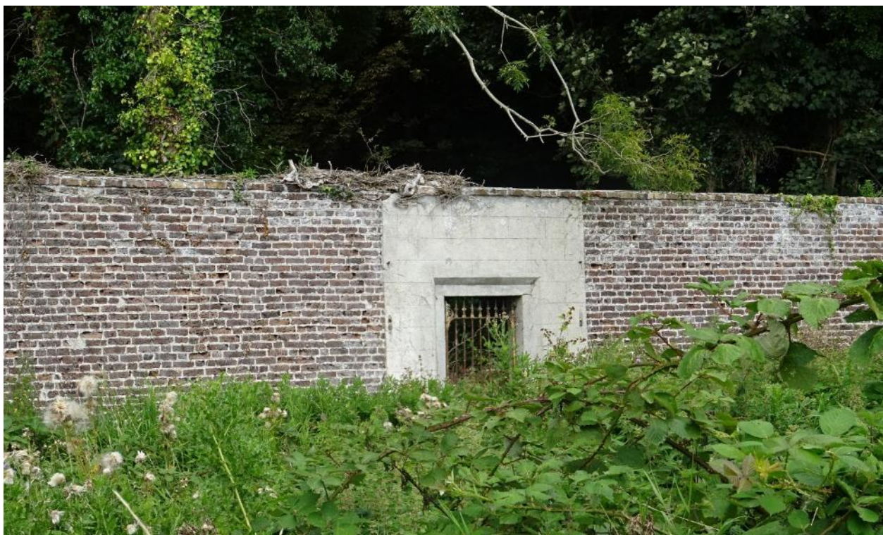
Fig.15: Section of protected north wall of Walled Garden, proposed for demolition.
